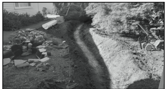
Figure 13. Channels can be excavated to accommodate landscaping features
