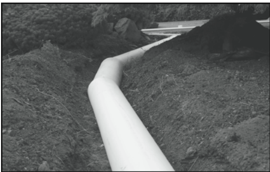
Figure 17. Cover the lateral pipe with half-pipe or low-profile chamber material
